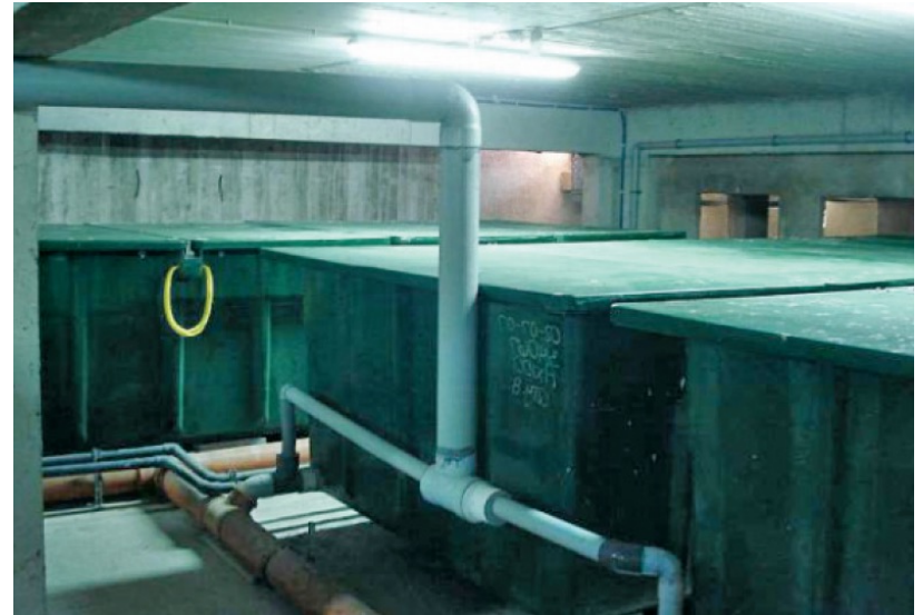
Underground Installation in Greece
